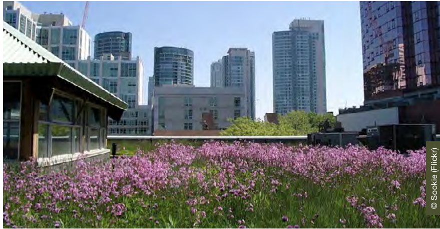
Toronto, Canada: Green roofs attenuate run-off offering mitigation to existing city drainage systems.
